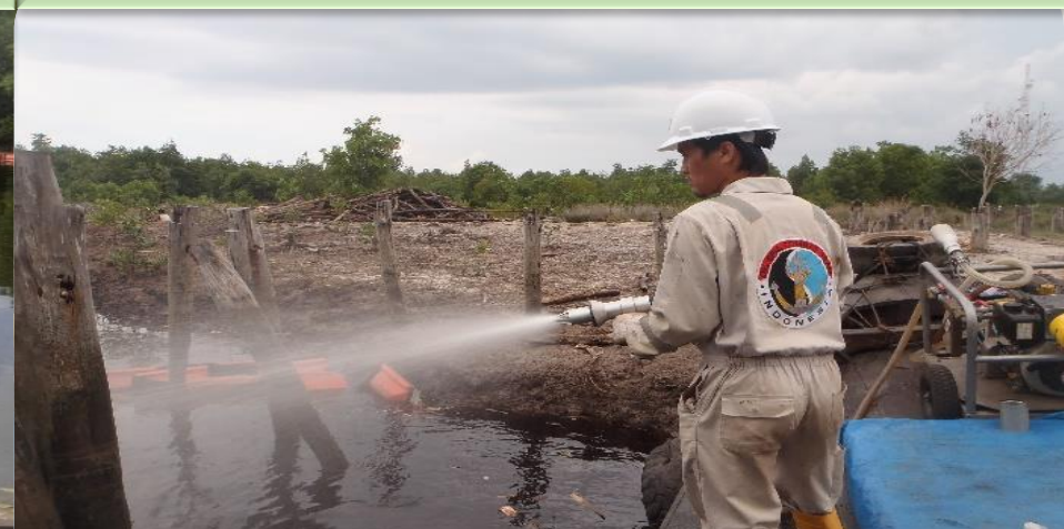
24 th of May 2014 Cleanup oil that sticks to vegetation using pressure hot water
