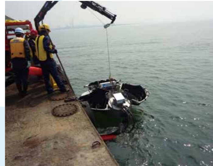
大型油回収機の投入(2号瀬戸内基地) Use of Large Skimmer (No.2 Seto Inland Sea Base)
