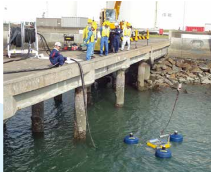
油回収機の投入 Use of Oil Skimmer
