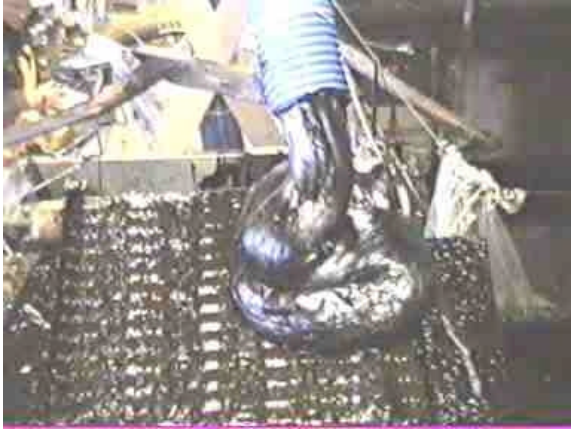
Figure 6 Cold bitumen, 33 m 3 /h @ 9 bar, 20 m discharge hose, injection is on but no water lubrication yet
