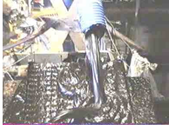
Figure 7 , Cold bitumen, 45 m 3 /h @ 2 bar, 20 m hose, water lubrication in full effect. Note the non sticky snake jumping up!
